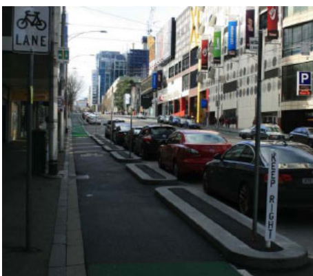
Path type: On-road separated cycle path Location: Melbourne, Australia Source: TMR, 2015
