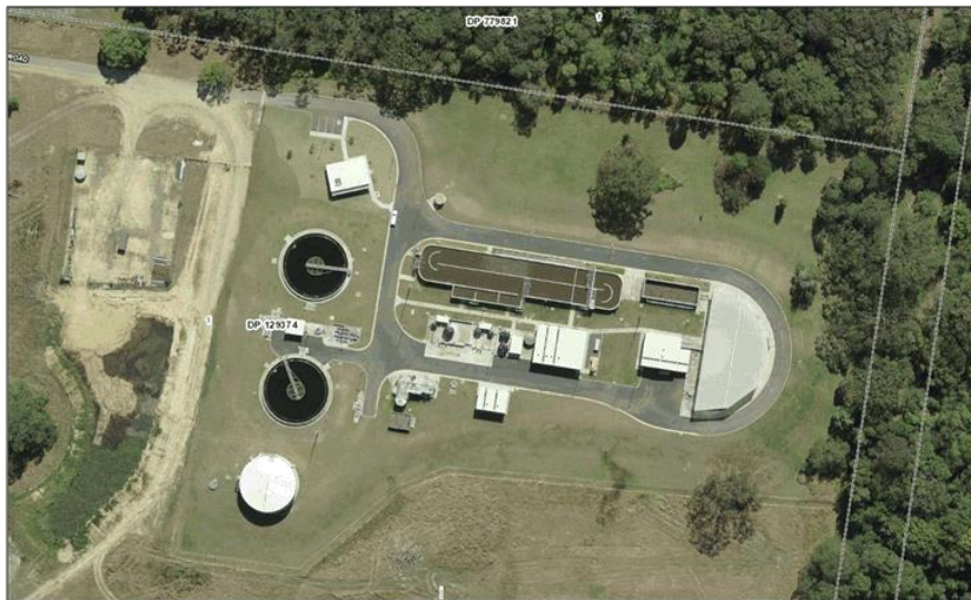
Figure 6 – Existing Sewage Treatment Plant area
