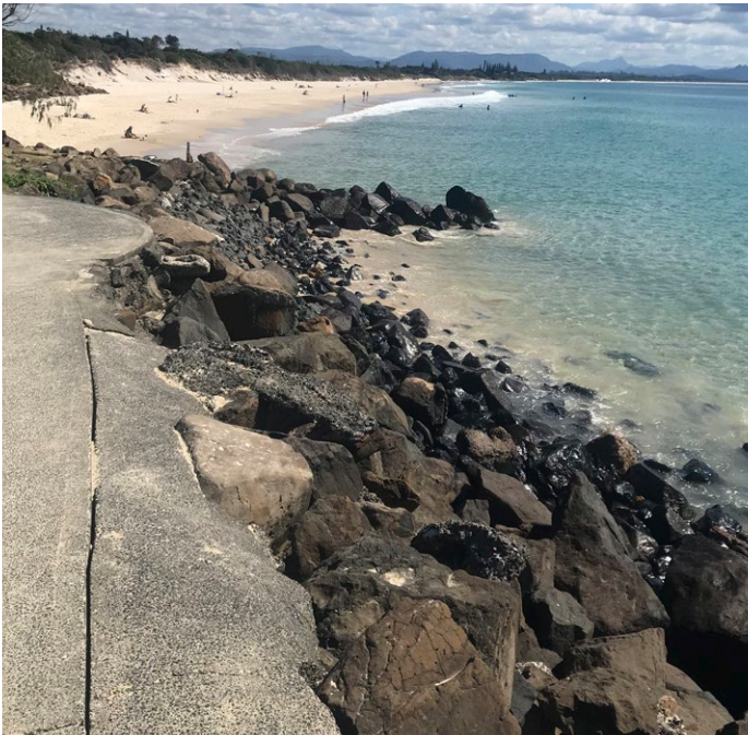
Existing rock protection wall- wall is degraded in places and presents safety issues for path users in some locations
