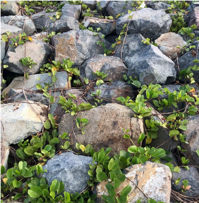
Basalt boulder infill
