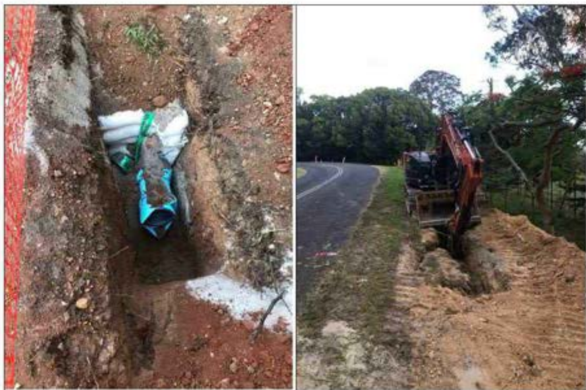
Plate 2-1 | Trunk water main pipe (DN400 HDPE) and construction machinery.
