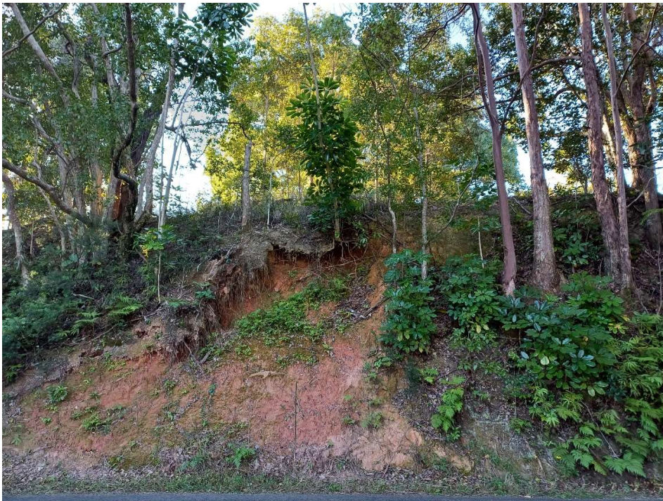
Figure 5. DM02303 upslope slip on northern embankment of The Pocket Road, Billinudgel 2483
