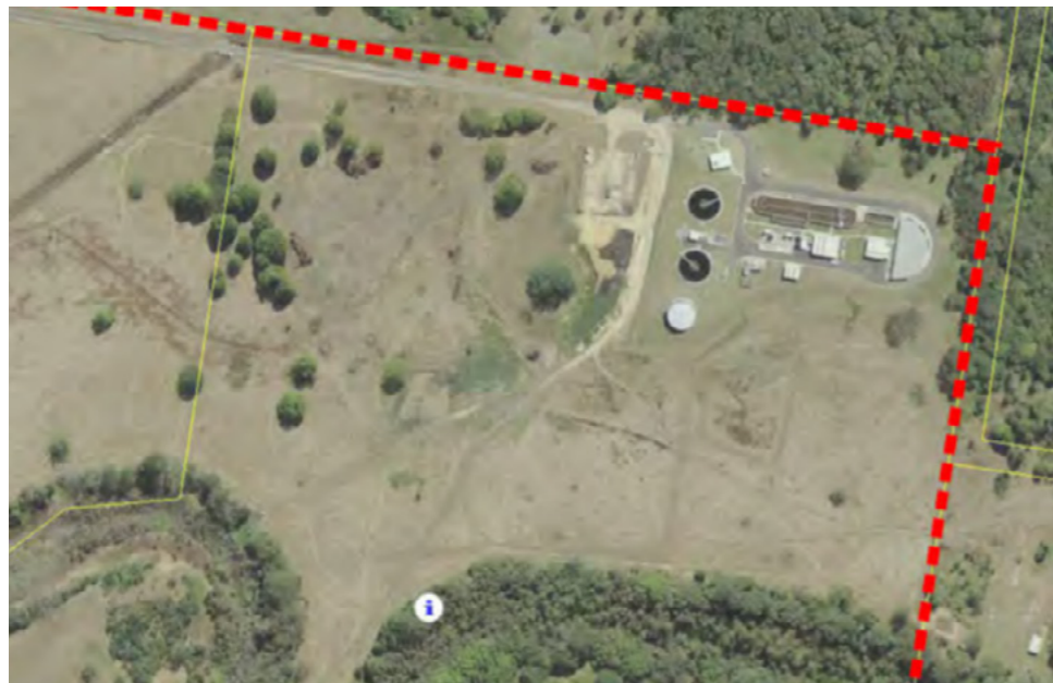
The existing BVSTP and the area to the west where the expansion is proposed.
