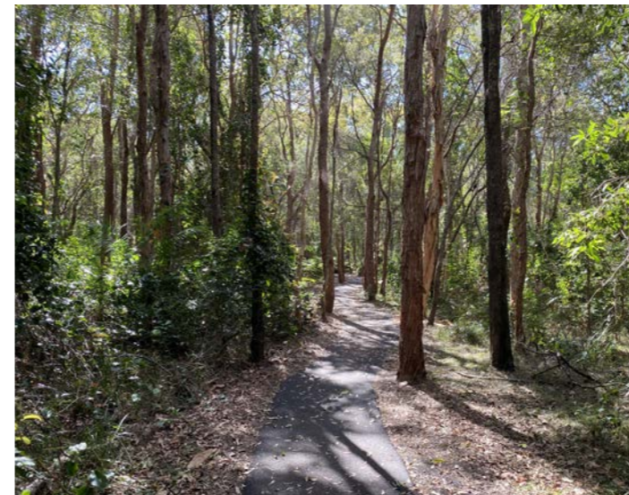
PATH SURFACES THROUGH ARBORETUM Accessible but flexible materials that require limited excavation and can be designed around tree locations- example images of walking tracks in Pottsville Environment Park and Daintree Rainforest
