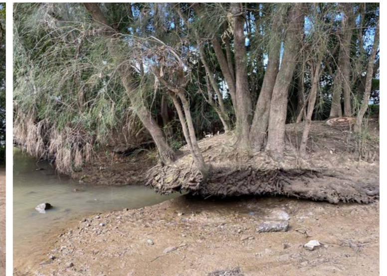
Existing significant erosion associated with the informal boat ramp in Heritage Park
