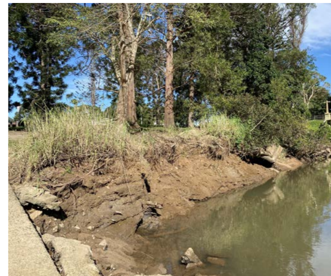
The Heritage Park West boat ramp is steep and under-utilised- adjacent riverbank areas are heavily eroded
