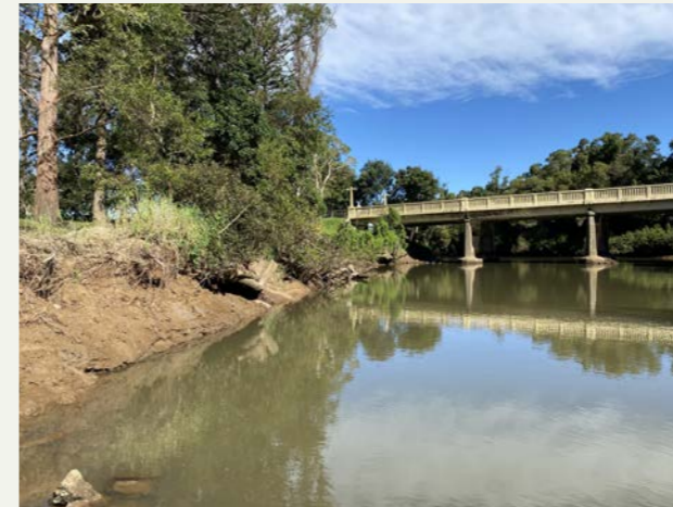
Riparian erosion stress
