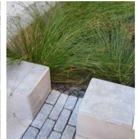
Paved channels with cut out in kerbs allow storm-water to be collected in rain gardens
