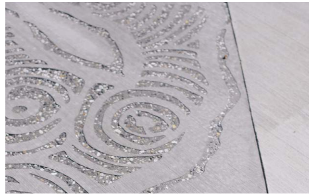
FEATURE TREATMENTS - CONCRETE PAVEMENT Potential to pattern feature concrete areas to highlight local creative talent- sandblast treatments or similar
