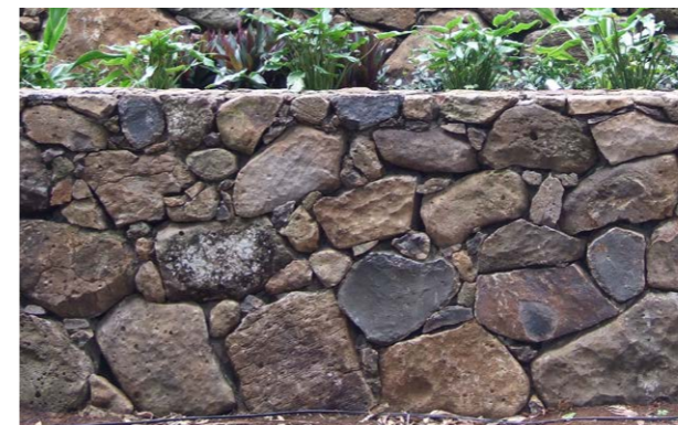
BASALT ROCK SEATING WALL Stone: Locally sourced basalt bush rock Joints: Coloured mortar joints Height: 450mm Width: 450mm
