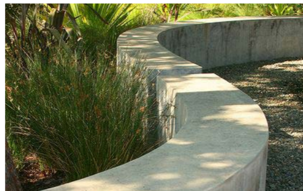
CONCRETE SEATING WALL Colour: Natural Grey Finish: Off form Height: 450mm Width: Varies
