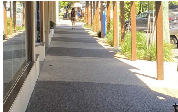
FOOTPATH - CONCRETE PAVEMENT Colour A: Belongil White Colour B: Woody Head Brown (Coomera) Finish: Lightly Exposed Pattern: 'wave' to match existing
