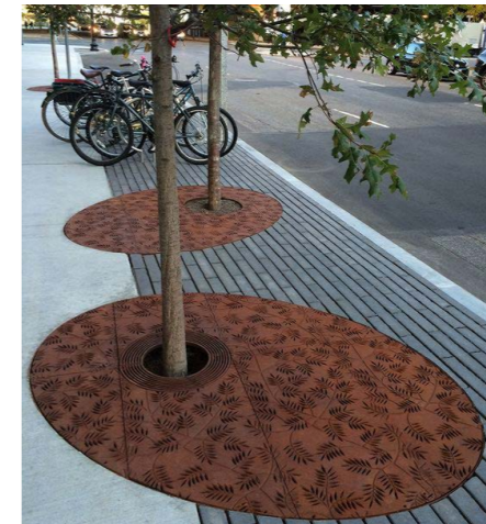
Tree grates implemented to allow full width pavements while storm-water is captured to water
