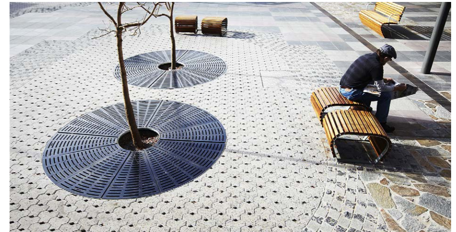
Permeable paving used to allow trees to be watered by storm-water
