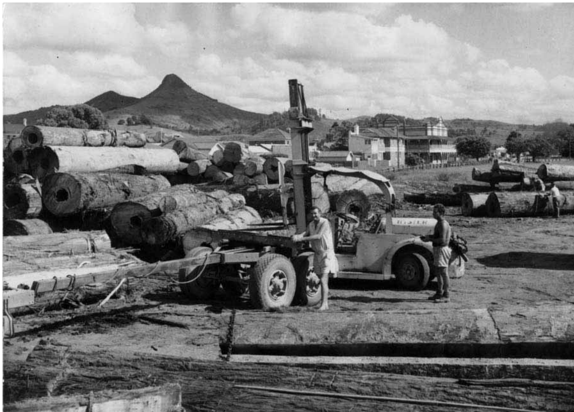
Figure 6: Log yards at Hollingworth's mill, Mullumbimby, c.1955. The Railway Hotel is in the right background ( Brunswick Valley Historical Society photo )
