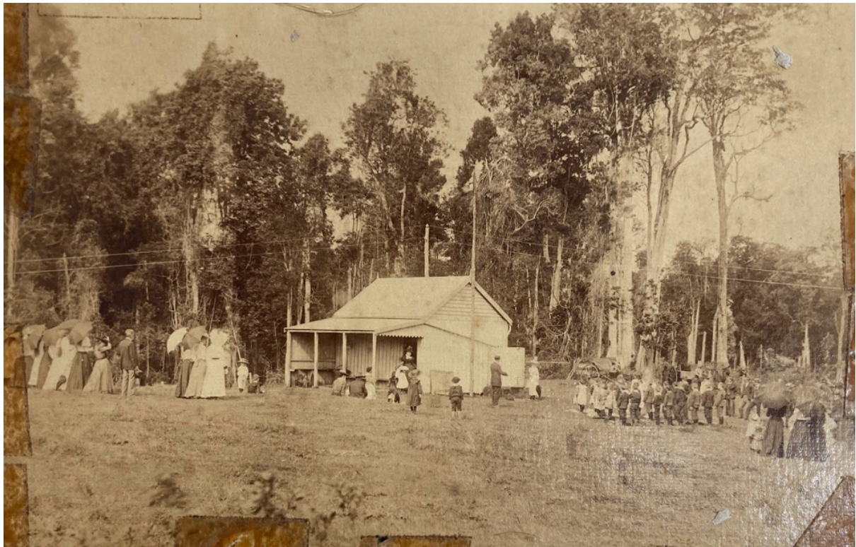
FIGURE 10: Jasper Public School, 1901. The original school was one 18'x15' room, with a 6ft verandah. All of the timber was pit-sawn from local trees. The building was demolished in 1943. Source: Richmond River Historical Society.
