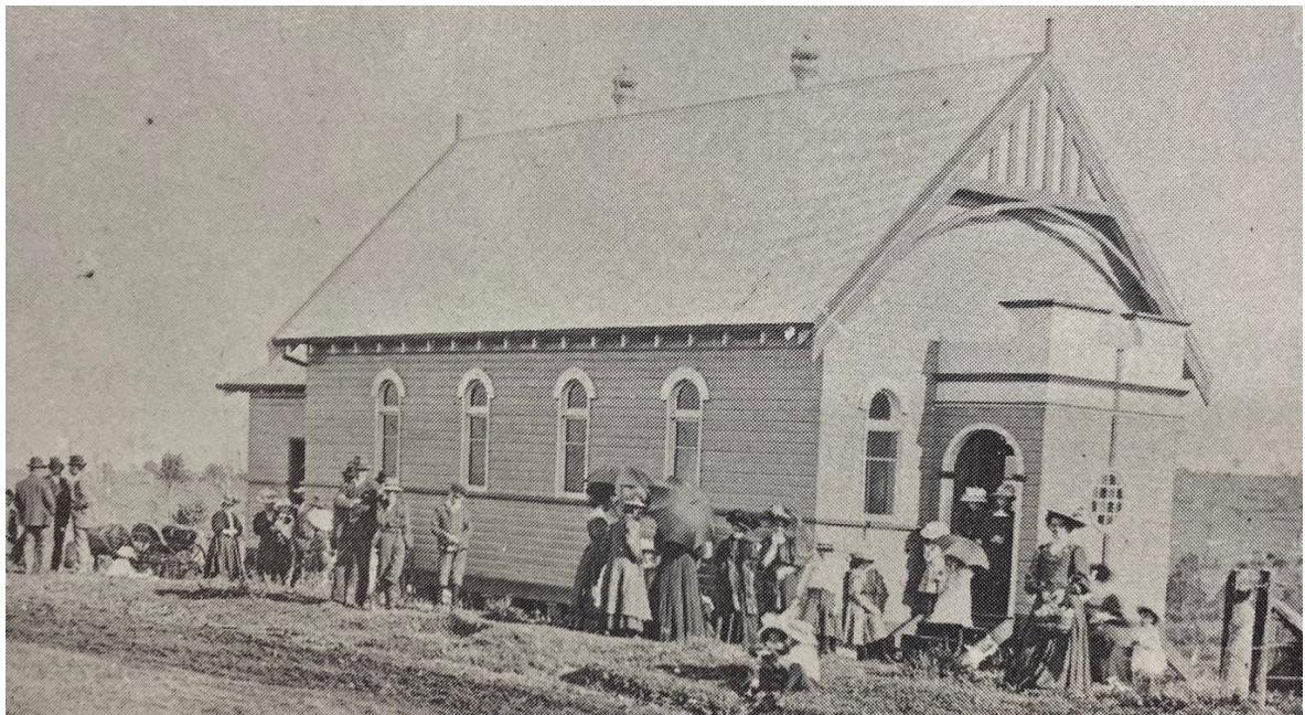
FIGURE 18: Methodist Church, opened in 1909. It was badly damaged in a storm in 1960 and demolished. Source: Centenary of Federal 1882-1982
