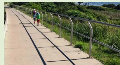
HANDRAIL/BALUSTRADE Material: HDG steel
