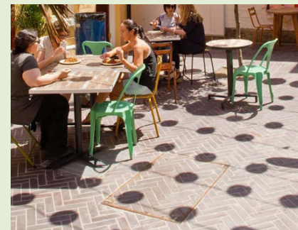
PIT LIDS TO MATCH ADJACENT PAVEMENT
