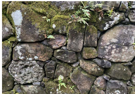
SEATING/RETAINING WALL Material: Locally sourced bushrock/basalt
