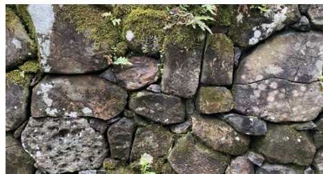
SEATING/RETAINING WALL Material: Locally sourced bushrock/basalt
