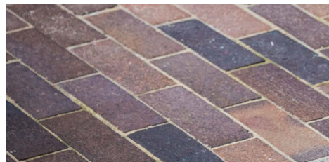
FOOTPATH FEATURE - BRICK FEATURES Type: Blue Mottle Paver Size: 225x75x55 Pattern: various Supplier: Lincoln Brickworks
