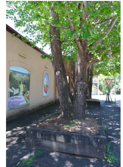
Existing timber retaining walls
