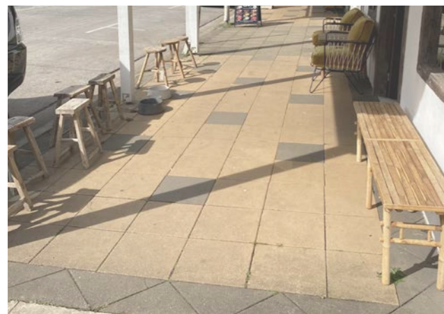
Concrete paving to shop frontage
