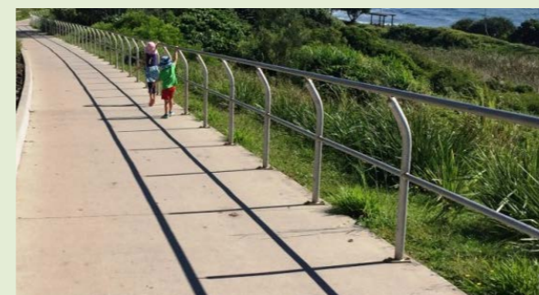
HANDRAIL/BALUSTRADE Material: HDG steel
