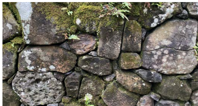
SEATING/RETAINING WALL Material: Locally sourced bushrock/basalt
