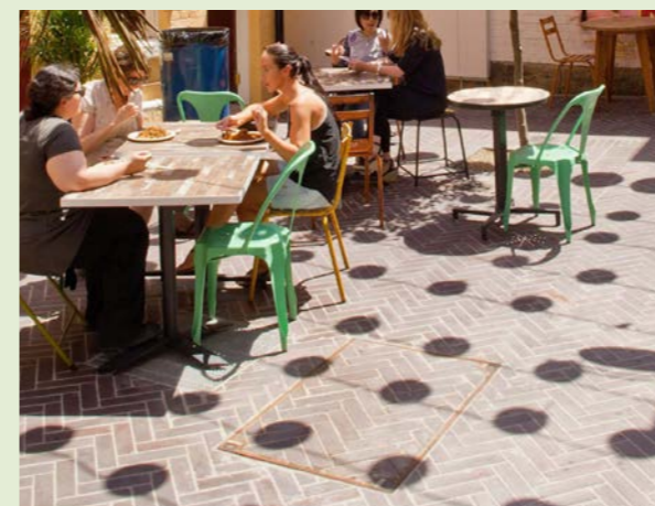
PIT LIDS TO MATCH ADJACENT PAVEMENT
