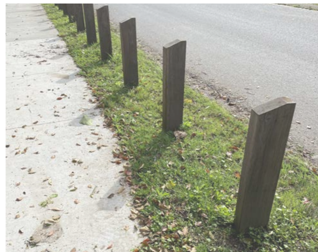
Hardwood timber bollards along Deacon Street
