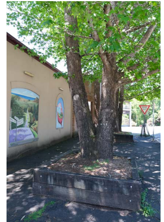
Existing timber retaining walls
