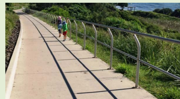
HANDRAIL/BALUSTRADE Material: HDG steel
