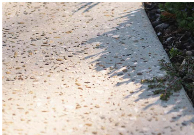
FOOTPATH - CONCRETE Colour: Wategos Exposed Finish: Lightly exposed Supplier: Holcim Geostone
