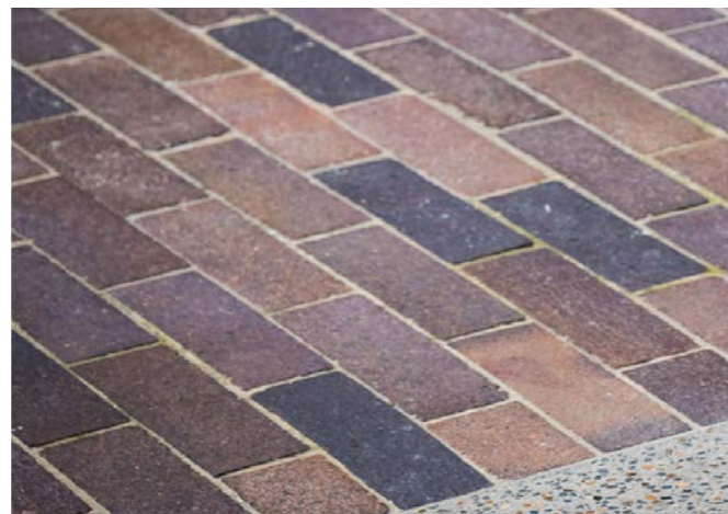
FOOTPATH - BRICK PAVING ON CONCRETE SLAB Type: Blue Mottle Paver Size: 225x75x55 Pattern: various Supplier: Lincoln Brickworks
