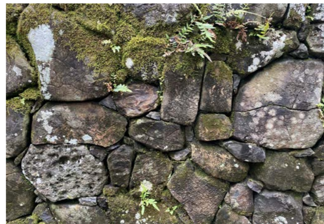
SEATING/RETAINING WALL Material: Locally sourced bushrock/basalt
