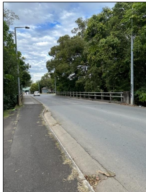
Photo 4 – Azalea Street bridge crossing adjacent to Jubilee Avenue
