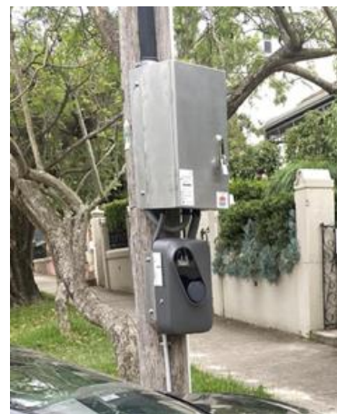
Pole Mounted Destination Charger
