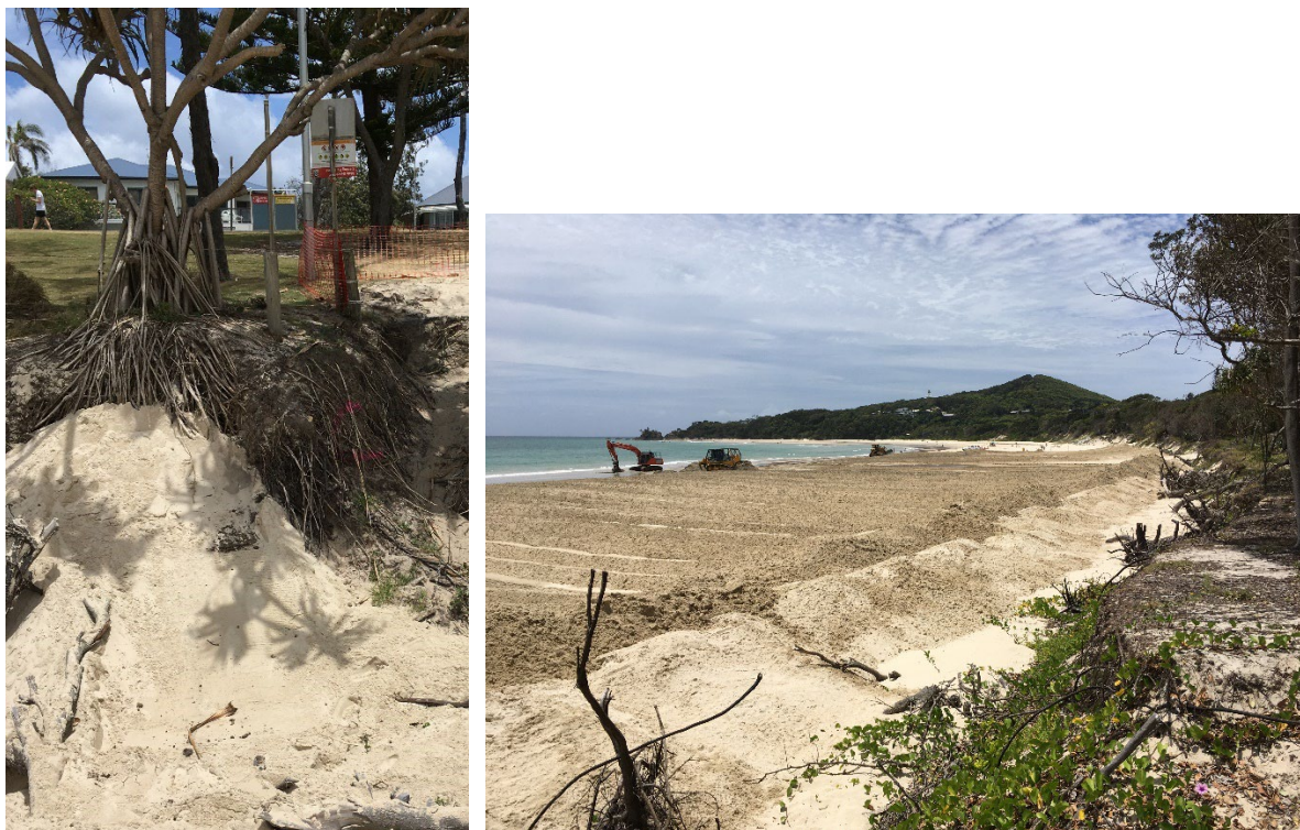
Figure 17: Sand pushed against the escarpment under exposed trees (left) and new incipient dune formation (right).
