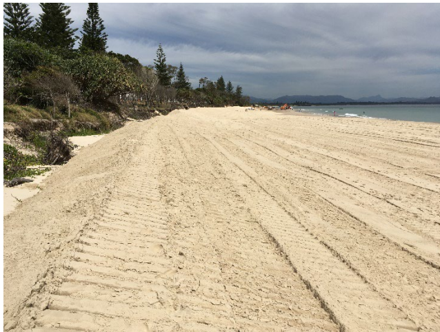
Figure 7: Newly built dune with machine tracks and machines in the background (left) and crab holes visible in machine tracks post-scraping works (right).
