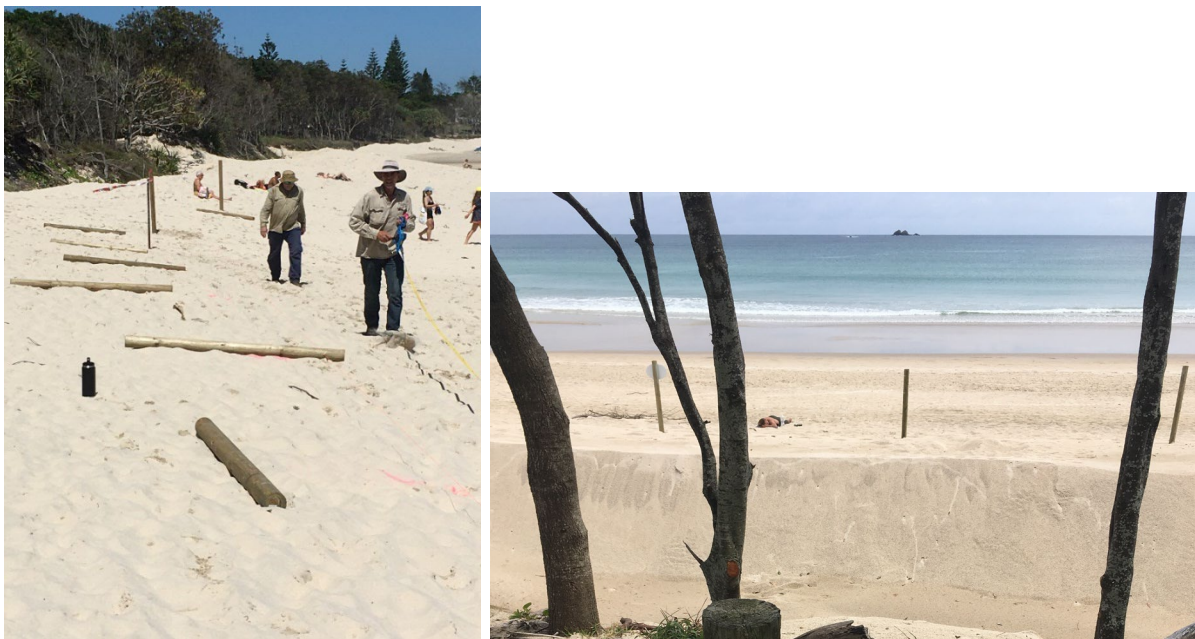
Figure 20: Fencing contractor - Clarkes Beach Café accessways (Access #11 from Figure 14) (left) and beachside fencing of Main Beach area (timber and 3-line wire) (right)
