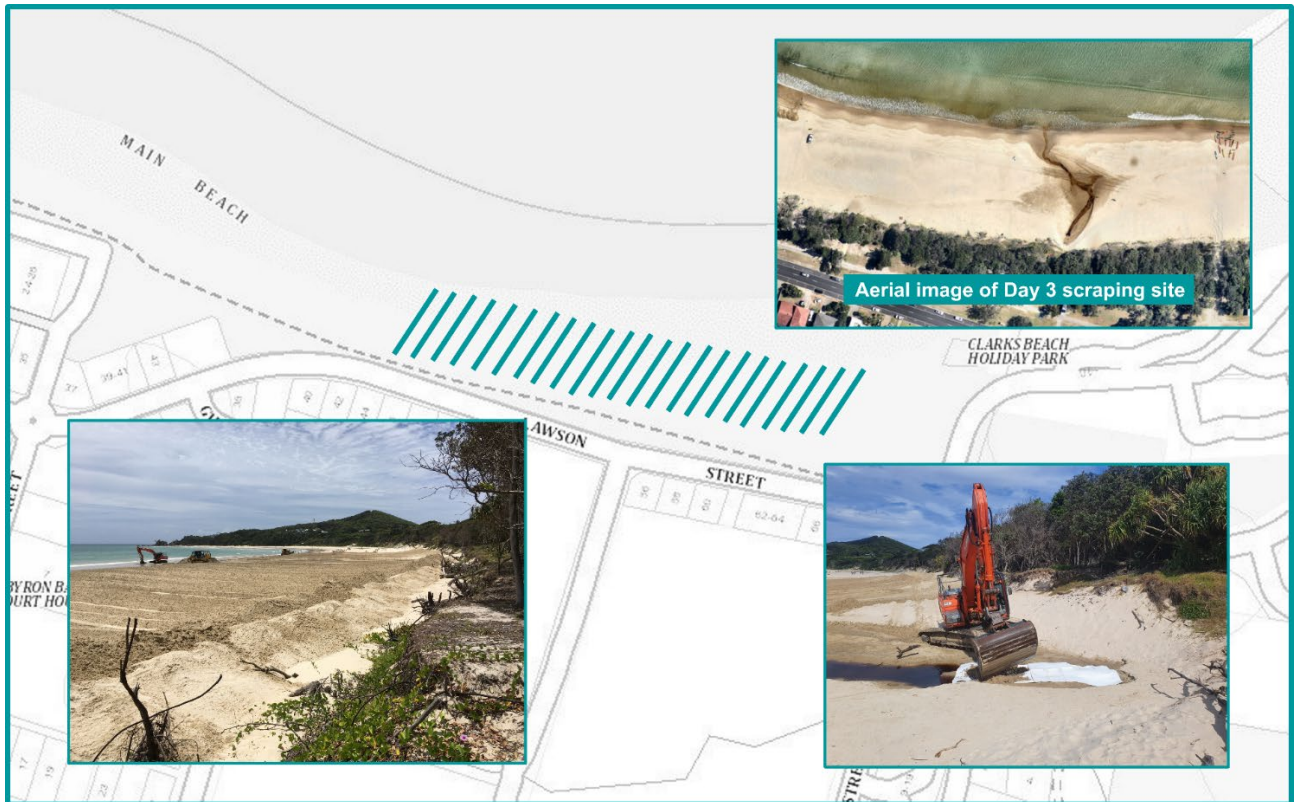
Figure 16: Day 3 (23/11/22) beach scraping works, located opposite 44 Lawson St to 62-64 Lawson St.
