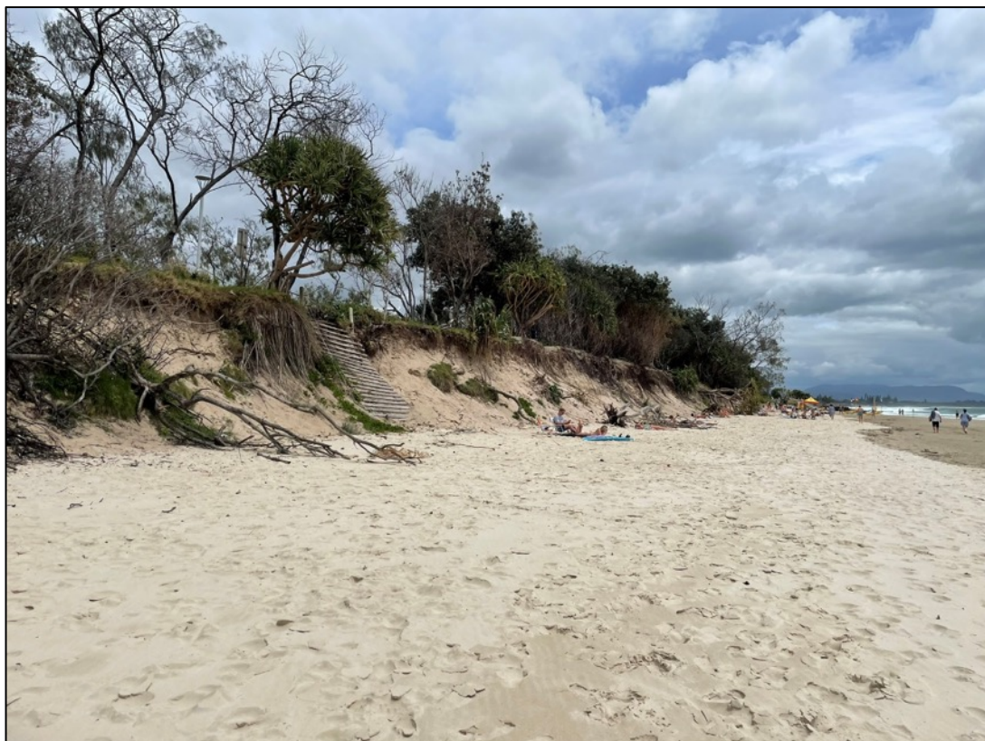
Plate 1: Dune scarping evident at the site.
