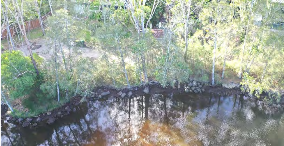
Plate 5: Scattered rocks along the bank indicating a previous revetment
