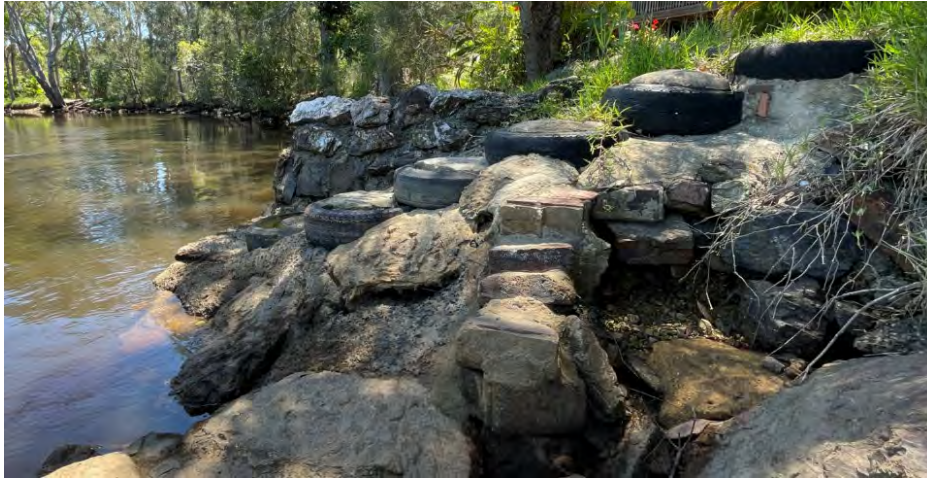
Plate 2: Inappropriate use of tyres, brick and concrete for erosion control and waterway access
