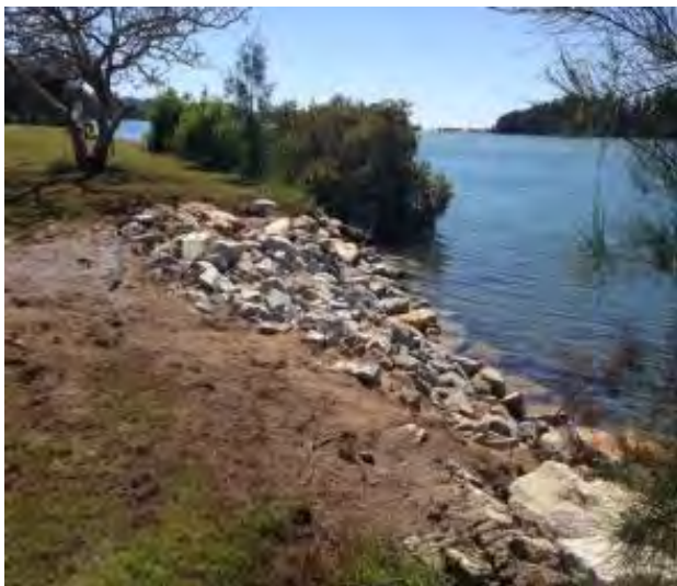
Plate 15: Example rock revetment
