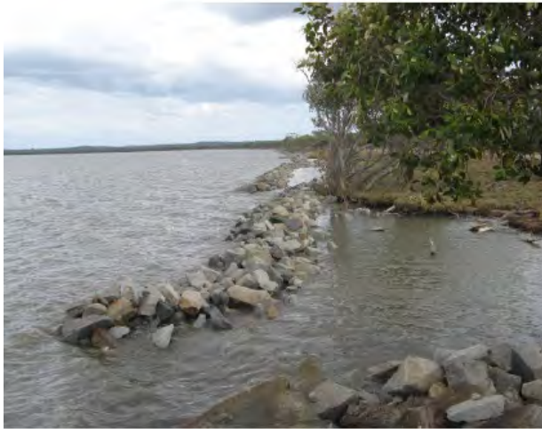
Plate 18: Examples of rock fillets
