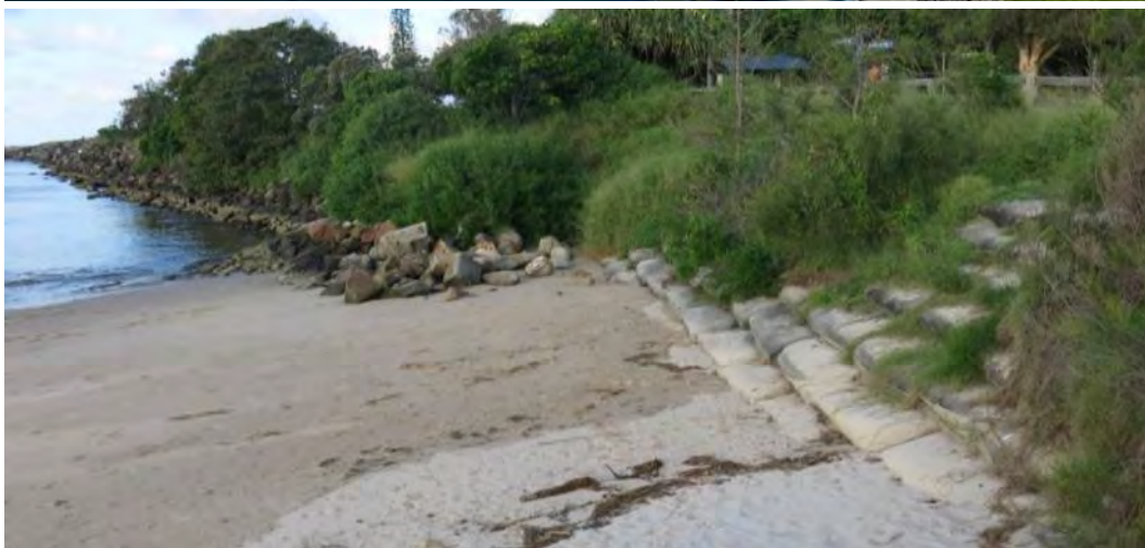
Plate 17: Example geotextile sand containers
