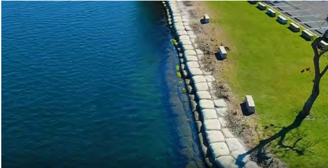
Plate 16: Example vertical seawall
