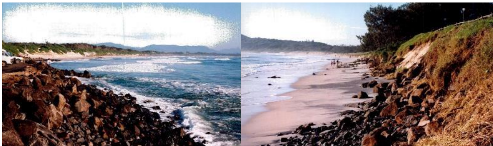
Figure 13: Photographs showing erosion (left) downdrift and (right) updrift of the JSPW in May 1999 (source: Peter Helman).
