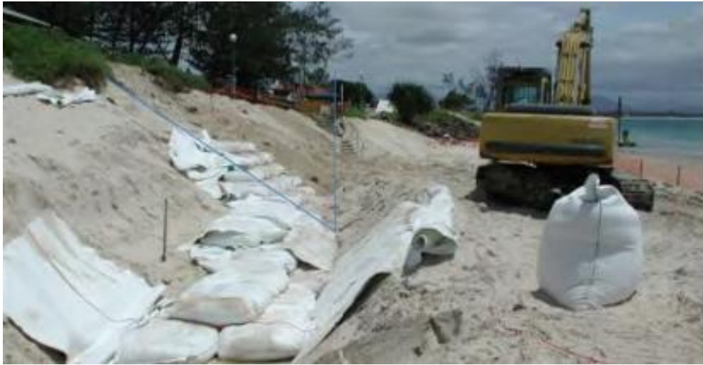
Figure 14: Photograph showing the construction of the interim geotextile revetment in front of the SLSC in 2002 (source: BSC).
