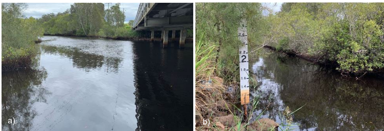
Plate 8: a) Belongil Creek at Ewingsdale Bridge b) Confluence of Butler Street Drain with Belongil Creek at Ewingsdale Bridge, note orange iron-staining at base of flood level marker.
