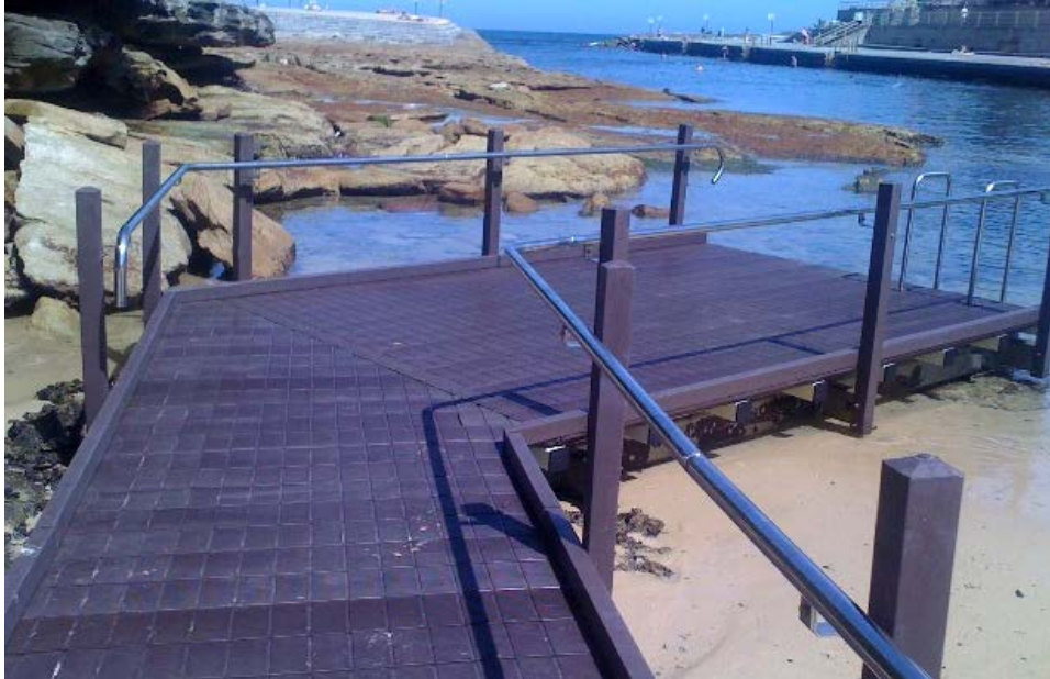
Example picture of recycled plastic walkway to a bathing area.
