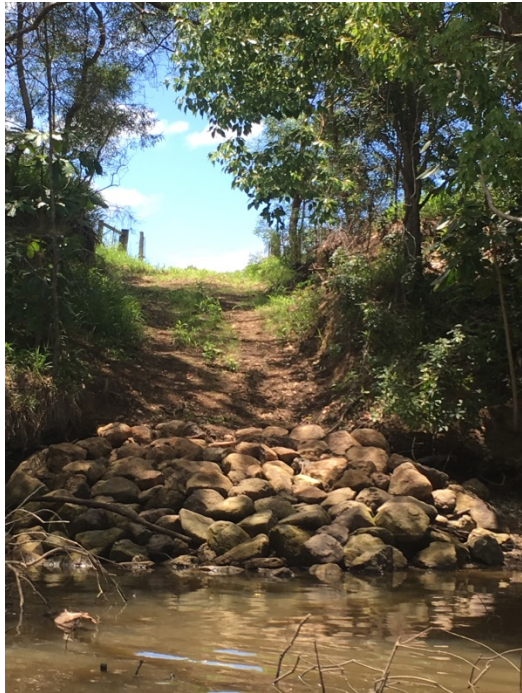
Photos – Site BR06 showing rock ramp revetment/pathway.
