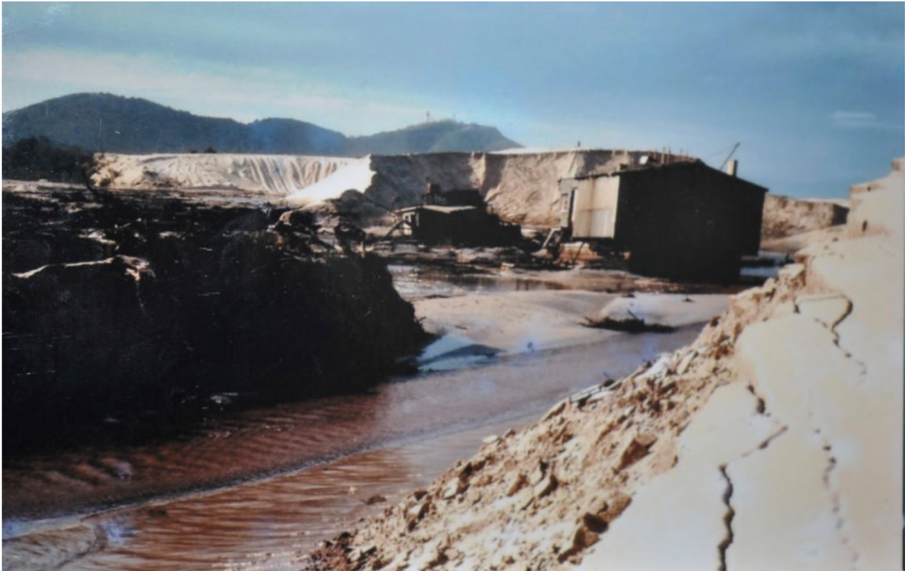
Figure E-3: Photo of dredge sand mining at Tallow Beach in the early 1960's, showing the Cape Byron lighthouse in the background (Source: http://byronbayhistoricalsociety.org.au/ )
