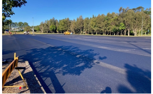
Photo: Resealing Cavanbah Centre car park
