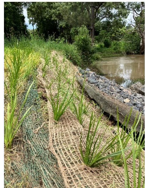
Photo: Works at an erosion scour hole adjacent the Brunswick River at Main Arm, completed through the River Rehabilitation Project.
