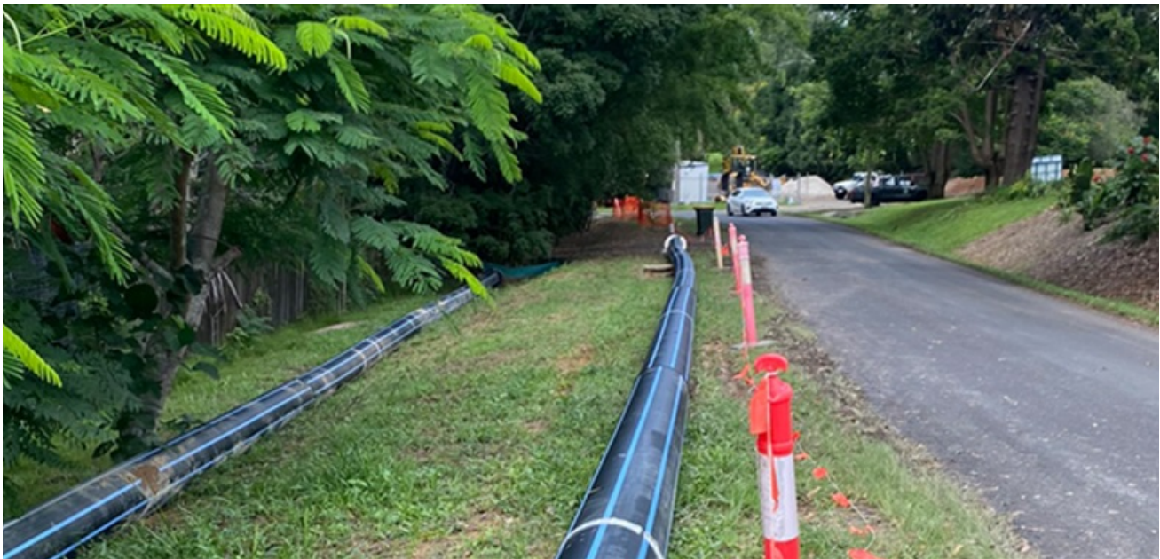
Photo: Pipe laying for Mullumbimby Emergency Water Main
