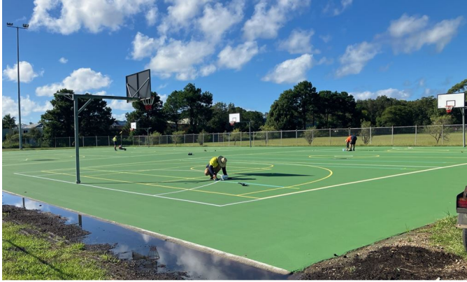
Photo: Cavanbah Centre netball courts repairs
