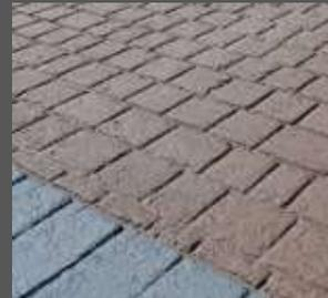
On-road threshold treatments to all entry/exit legs of the roundabout - consider stamped asphalt.
