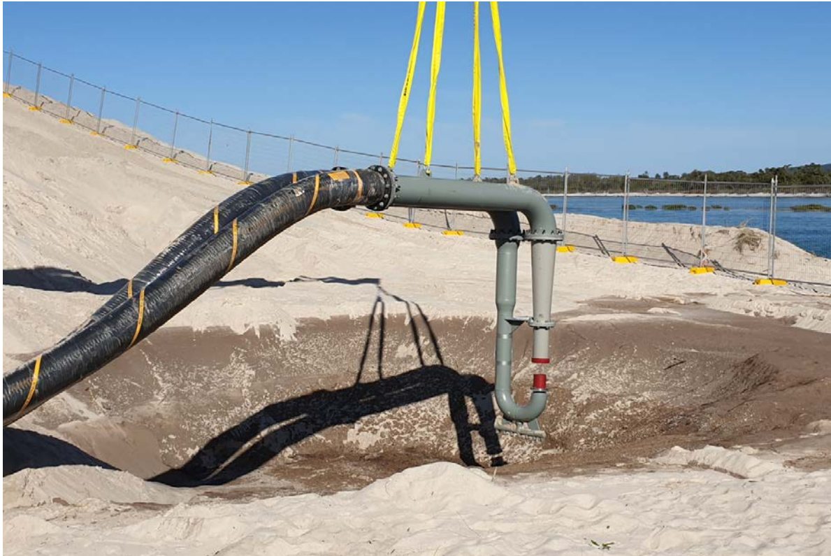
Figure 7: Photo of a jet pump being installed at Jimmys Beach.
