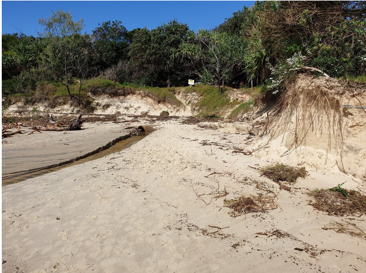
Figure 65: Dune erosion around stormwater outlet on upper beach at Clarkes Beach (photo taken July 2020).
