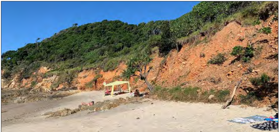
Figure 8: Looking west towards the headland showing slumping in the foreshore dunal system.
