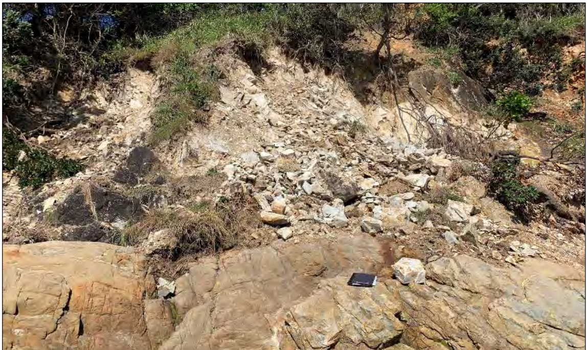
Figure 9: Looking south east towards a recent wedge-failure.
