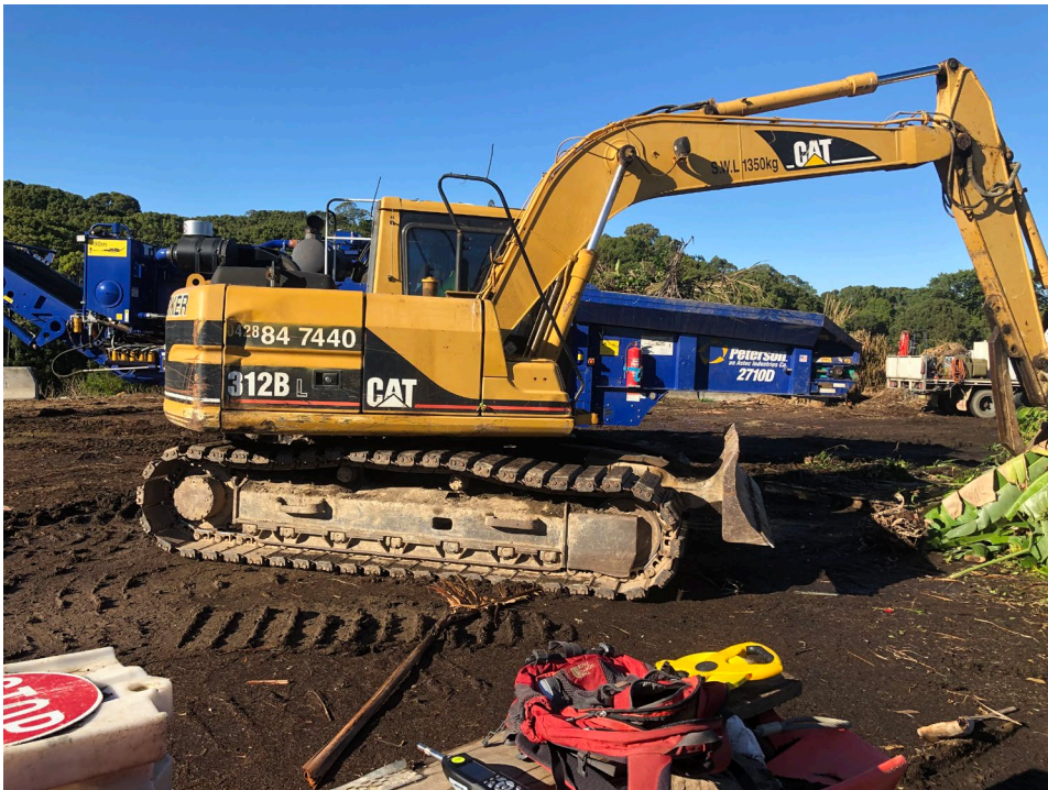
Photo B Excavator feeding Mulcher
