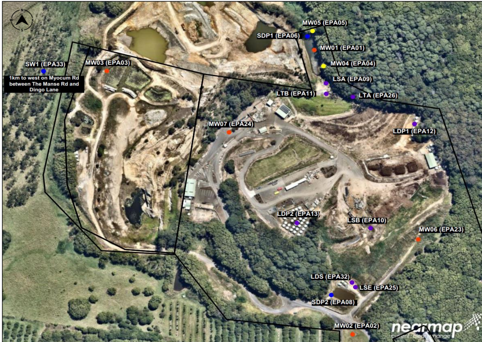
Figure 2-3: Myocum Landfill Monitoring Points (Image Source: NearMap 3 October 2021).
