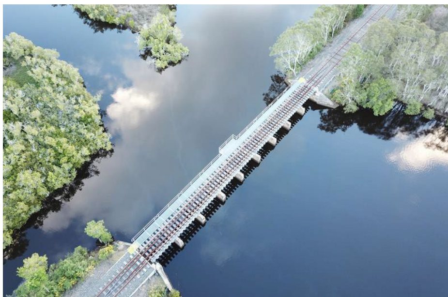
Figure 4.7: Belongil Creek Railway Bridge after restoration by Byron Bay Railway Company
