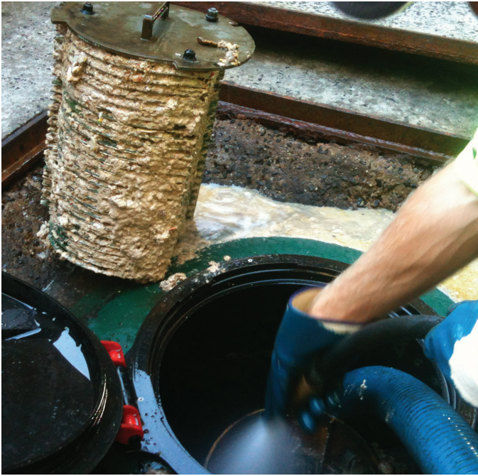
An overloaded grease arrestor overdue for service
