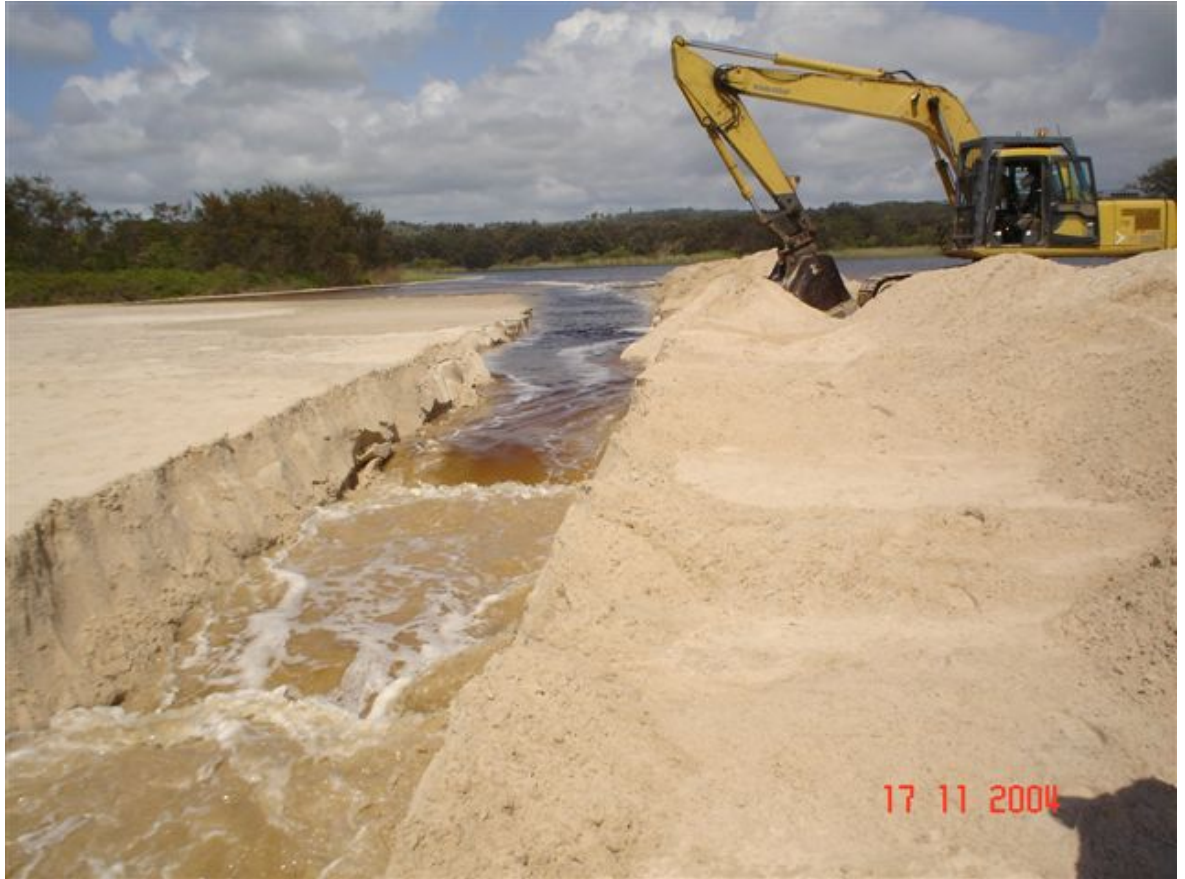
■ Figure 5-5 Manual opening of Tallow Lake mouth to relieve flooding, November 2004
