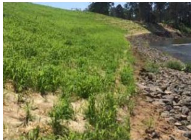
Figure 5: An example of river bank rehabilitation at Mockers Road, Fernvale. This image was sourced from the Mid-Brisbane Catchment Action Plan delivered by the Council of Mayors (SEQ) Resilient Rivers Initiative.
