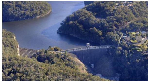
Figure 8: The Nepean Dam in New South Wales. This image was sourced from WaterNSW.
