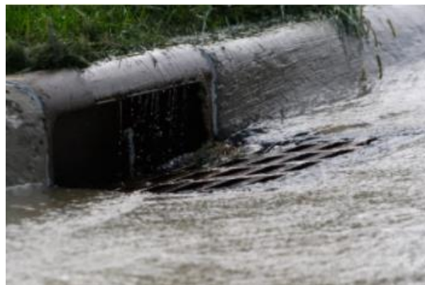
Figure 9: This figure shows stormwater flowing into the stormwater drainage network. This image was sourced from the City of Shoreline in Western Australia.
