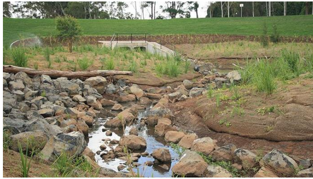
Figure 6: The detention basin at Garnett Lehmann Park, Toowoomba. This image was sourced from ABC Southern QLD and was photographed by David Illiffe.
