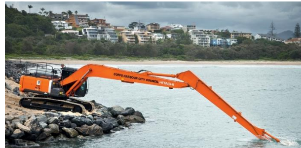
Figure 7: Dredging at the mouth of the Coffs Harbour boat ramp. This image was sourced from the Hitachi website.
