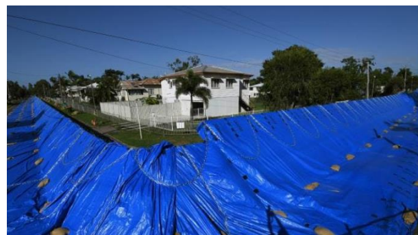
Figure 3: Temporary levee in Rockhampton. This image was sourced from the Courier Mail and was photographed by Dan Peled.
