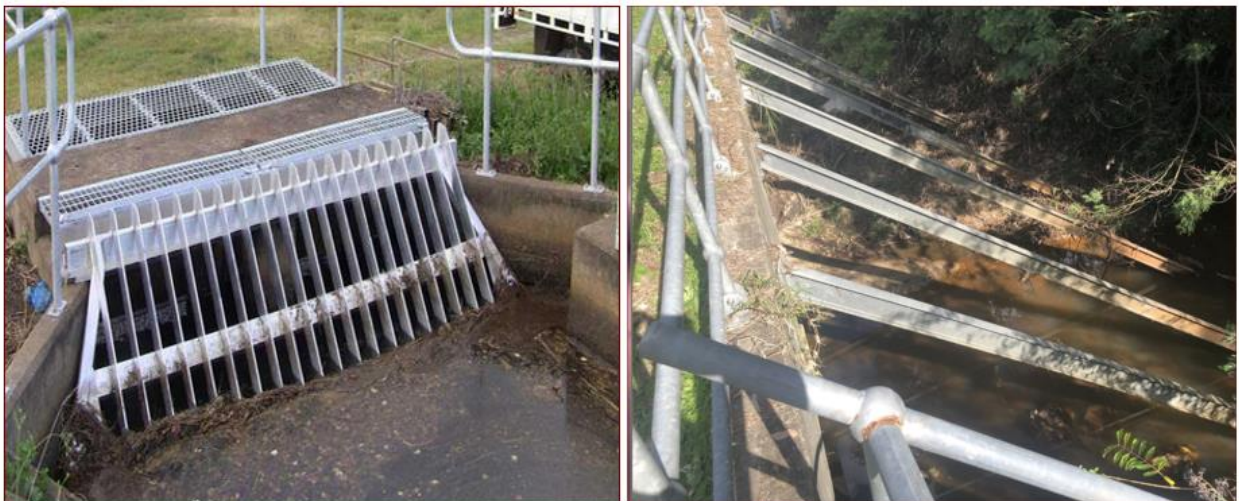
Image 1: Examples of structures to reduce blockage of a culvert and pedestrian bridge.
