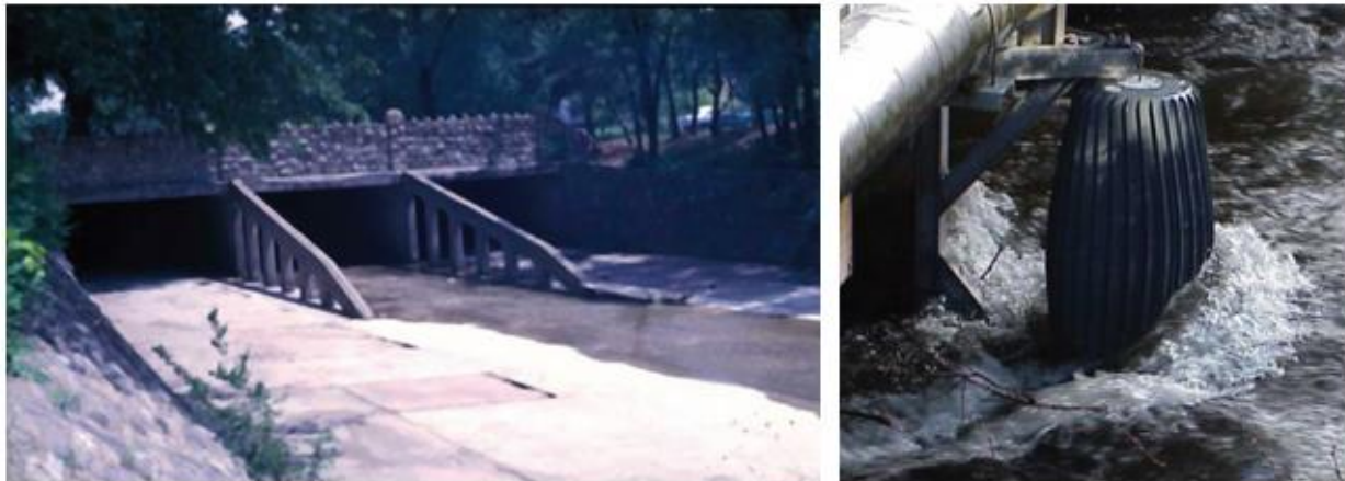
Image 2: Examples of debris control measures for large hydraulic structures. Left – example of debris fins. Right– an example of a debris sweeper (2005, US Department of Transport Federal Highway Administration).
