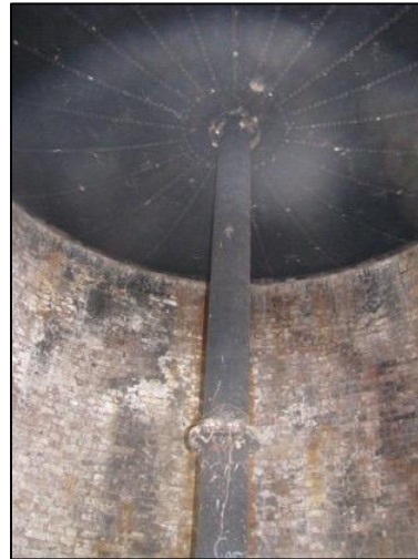
Figure 122: Interior of Meranburn Water Tank (Source: Image by BJ Hickson, NSW Heritage Inventory)
