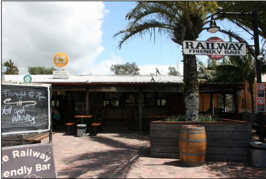
Figure 92: Large verandah addition to the eastern elevation. Weir Phillips
