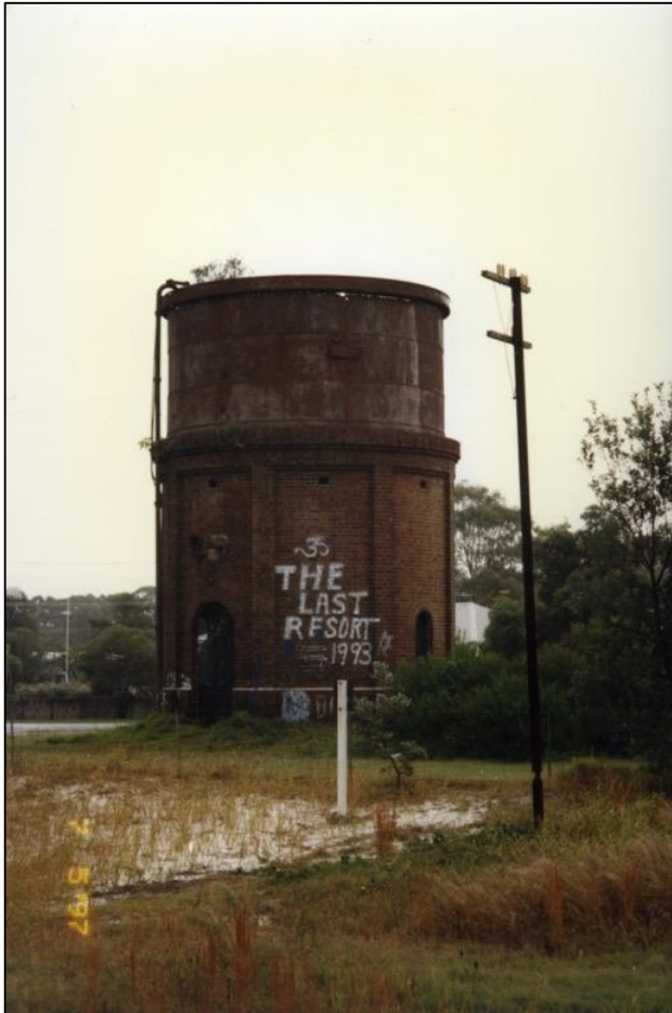
Figure 34 Water Tank with decorative base constructed by William Mitchell. Dunn
