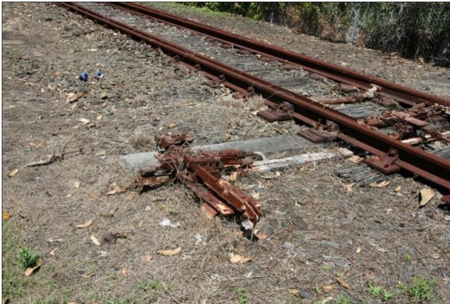
Figure 110: remaining components of railway switch. Weir Phillips
