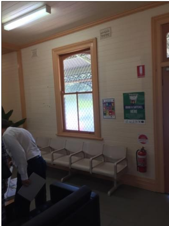
Figure 73: Original timber Sliding sash window. Weir Phillips
