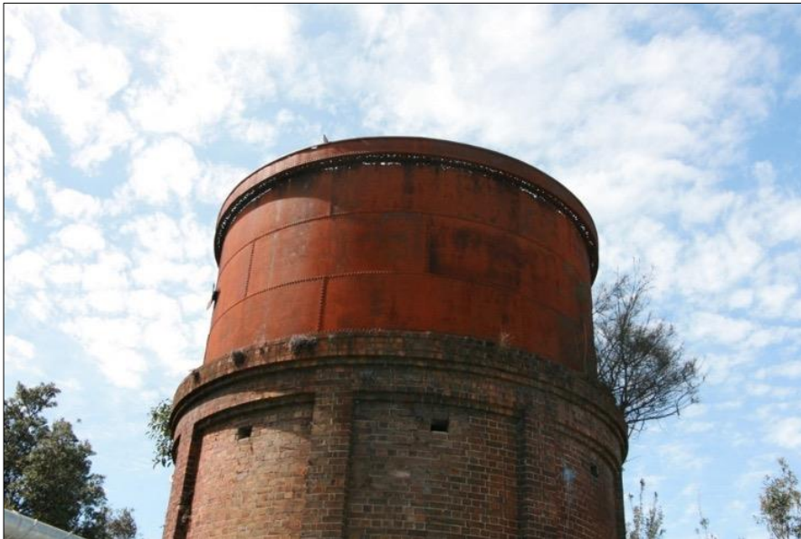
Figure 97 The tank is deteriorating. The corrosion has formed holes beneath the upper rim. Weir Phillips
