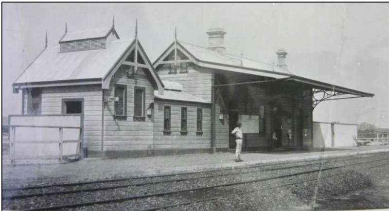
Figure 27: Undated image of Byron Bay Station. Note that the tracks are level with the platform and not in a cutting as currently shown on site. ARHSnsw
