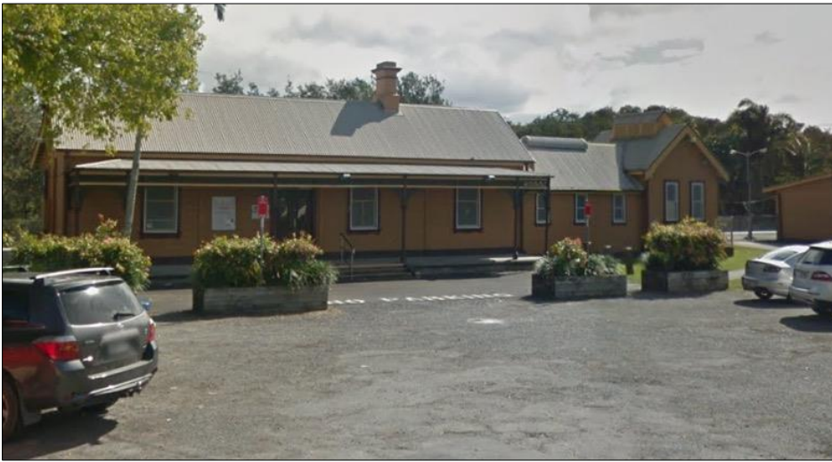
Figure 66: Former Railway Station Building as viewed from the East. Google Maps.
