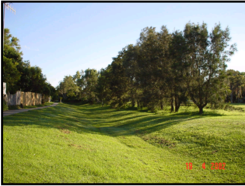
Figure B9.8 – Example of drainage line that encourages the use of natural materials. Note: Planting species should be tolerant of inundation and not likely to create a weed problem.
