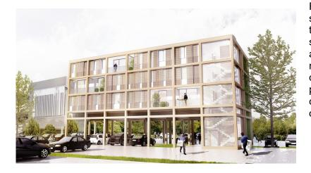
Finally, the planning for this multistorey residential building is transferable to other plots. The supporting structure allows adaptable floor plans in all three residential floors, which can be divided individually via light partitions. The supporting structure consists of composite floors made of wood and concrete.
