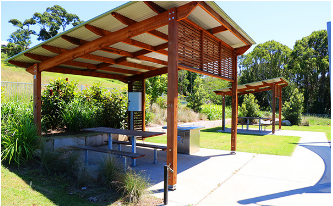
Figure 3: This photo shows the existing picnic shelters adjacent to the play space.
