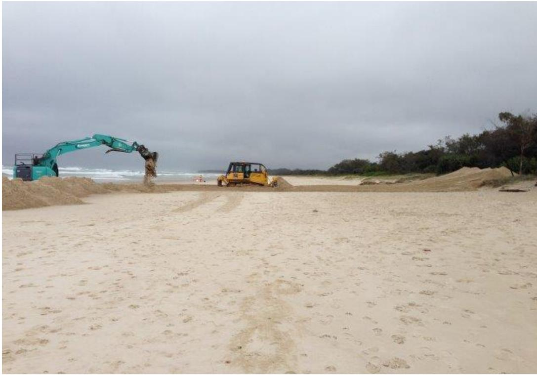
**Figure 19: Excavator working in the intertidal zone building sand piles; bobcat pushing sand onto the dune face (New Brighton, October 2017).**
