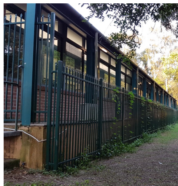
Plate 8.5 View east between the courthouse and the northern side of the flying-fox camp
