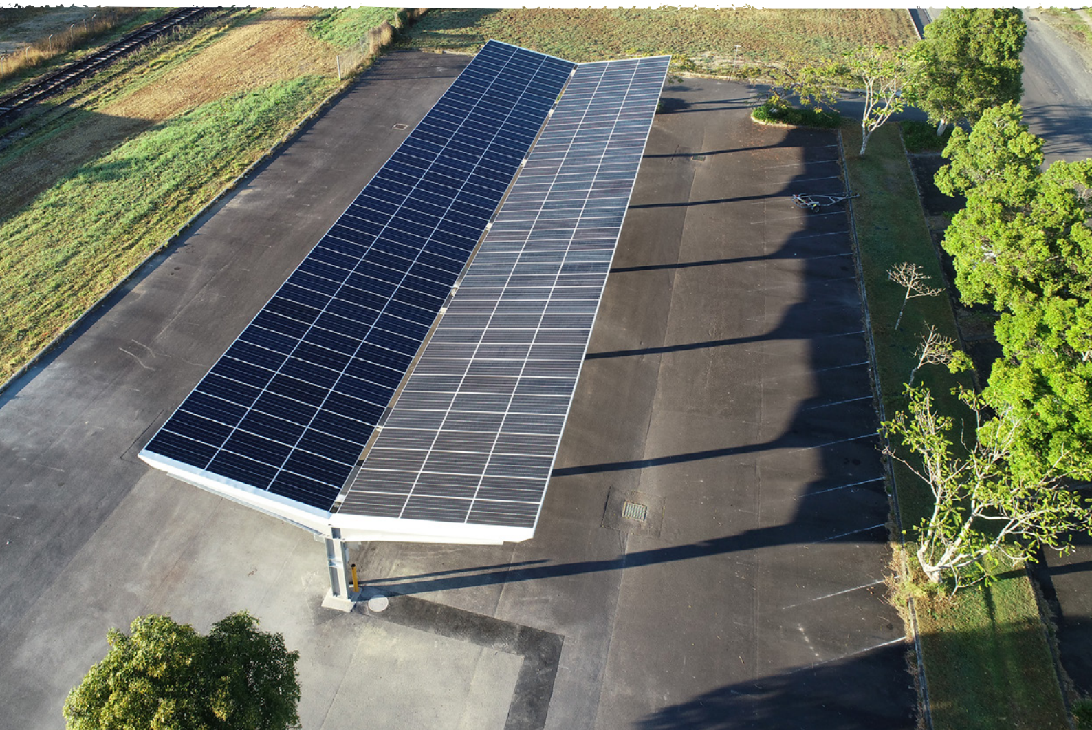
The 99 kW solar carport structure at the Council Administration Building, Mullumbimby
