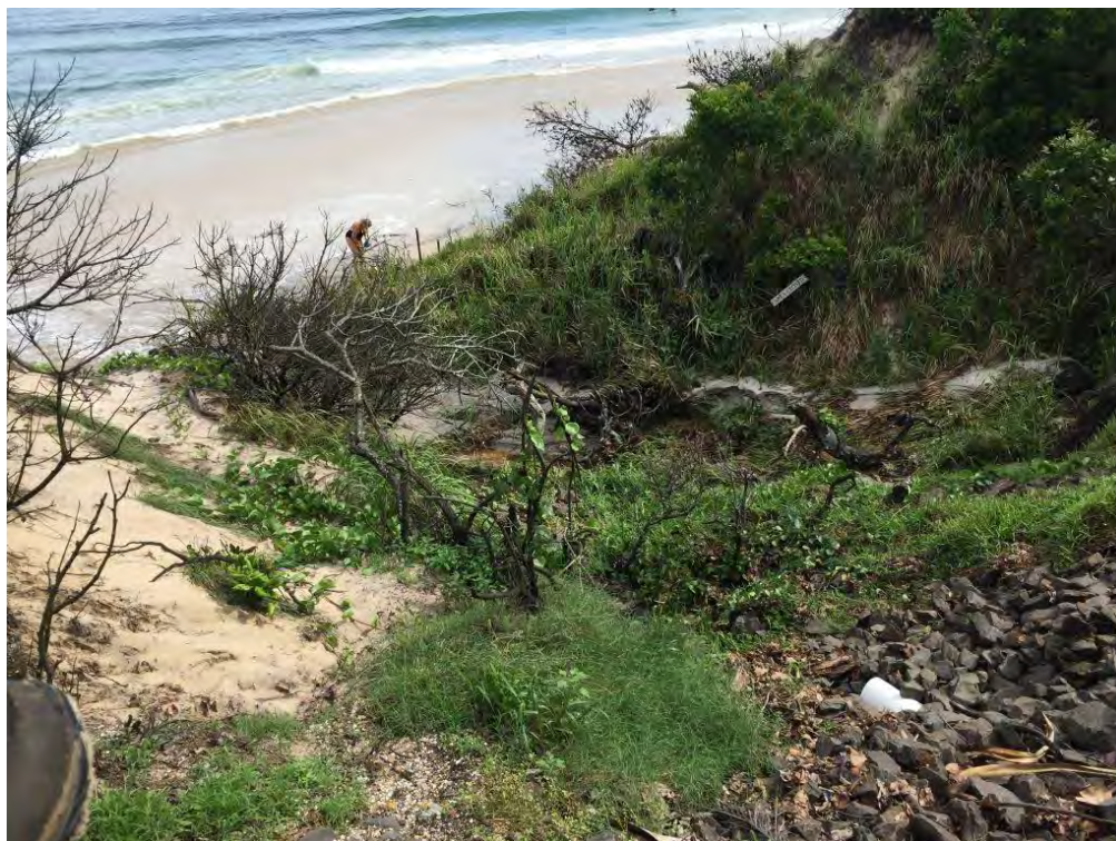
Figure 3-7 Eroded gully at eastern end of Reflections Holiday Park
