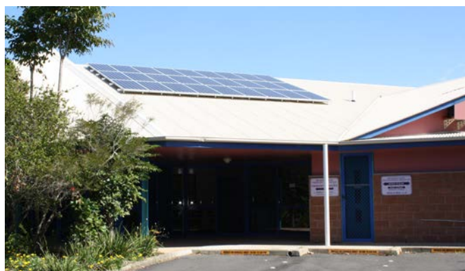
Solar panels on the Brunswick Heads Community Centre reduce greenhouse gas emissions by supplementing the centre's energy use with electricity made from the sun.
