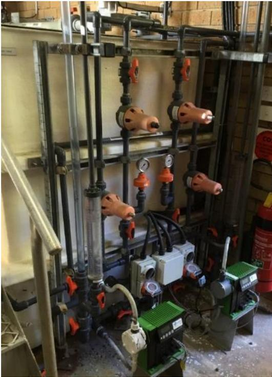
**Figure 6** Chemical dosing pumps
