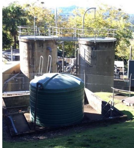
**Figure 3** Chemical dosing and flocculation chambers
