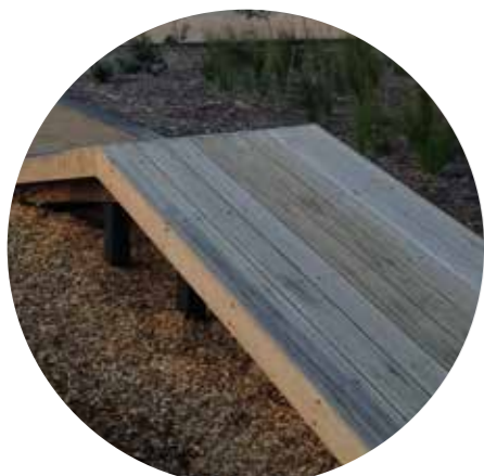
Elements ramping over trunks
