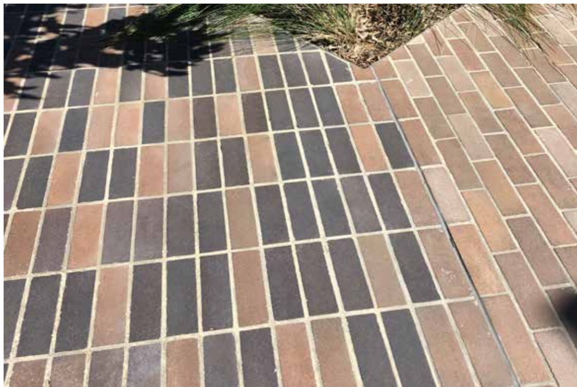
Brick paving- feature pavement for circuit / apron to central circle timber element
