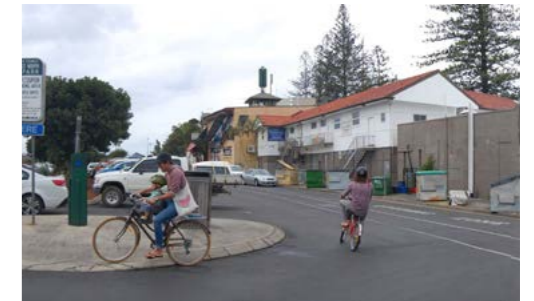
Figure 5.10 - Existing view of Lawson Street Car Park
