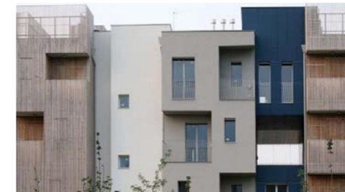
Roof articulation varies street frontages.
