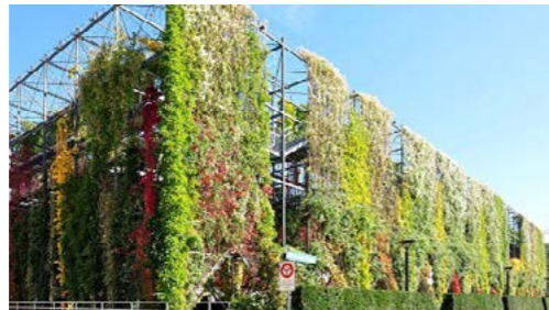
A plant covered Multi-Storey Car 'PARK' facility.
