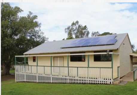
Scout Hall entrance and verandah
