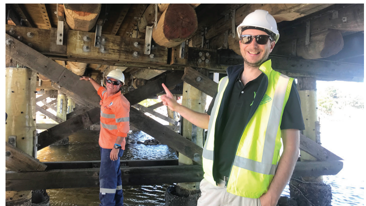
Engineer Josh Provis underneath the Brunswick Head Bridge
