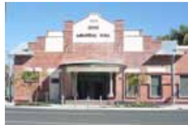
Mullumbimby Civic Memorial Hall 55 Dalley Street Mullumbimby (Board of Management)
