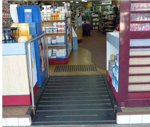
Mullumbimby Chemist – clear path of travel from outdoor to indoor areas, handrail and tactile surfaces
